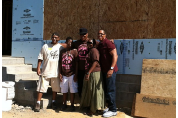
Mark Neal, future owner of the Sweet 16 house, and family have already put a lot of sweat equity into building Mark's home.
