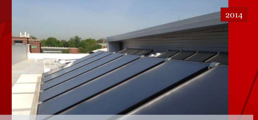
In spring 2014, UofL installed a 16-panel, 165 MMBtu solar pool heating system on the roof of the Ralph Wright Natatorium to tackle the high energy demands of regulating the temperature of the largest body of water on campus - our Olympic-size pool!
