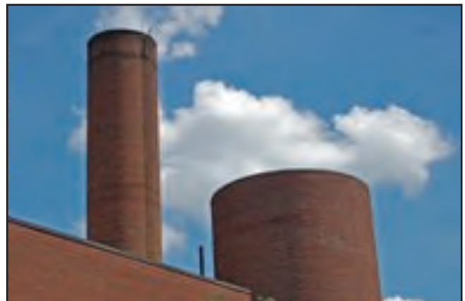
Belknap's steam & chilled water plant is transitioning away from coal to 100 percent natural gas by 2015.
