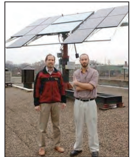
Researchers installed a dual-tracking solar PV array on the roof of Sackett Hall at the J.B. Speed School of Engineering.
