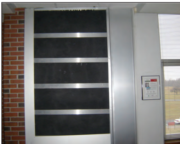
An experimental passive solar heat tube for warming classroom space is being studied at Burhans Hall on Shelby Campus.
