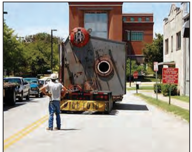
In July 2010, UofL sent an old coal-fired boiler to a nearby recycling facility to make room for a more efficient natural gas boiler at the Belknap steam and chilled water plant.
