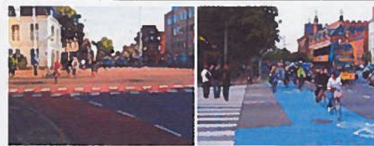
F. Colored bike lanes are used in many cities to improve visibility and so car drivers can better understand bike travel zones.
