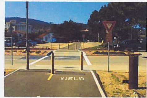
Bike and pedestrian crossings of vehicular traffic zones should be clearly marked to prevent car access and warn cyclists and pedestrians.
