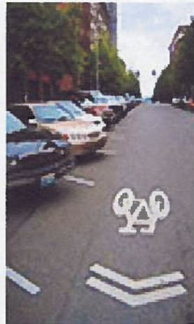
E. Sharrow Bike Lane and back-in, diagonal auto parking spaces improve visibility.
