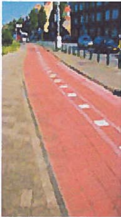
D. Surfaces to clearly define separate bike and pedestrian zones on off-road mixed use pathways.
