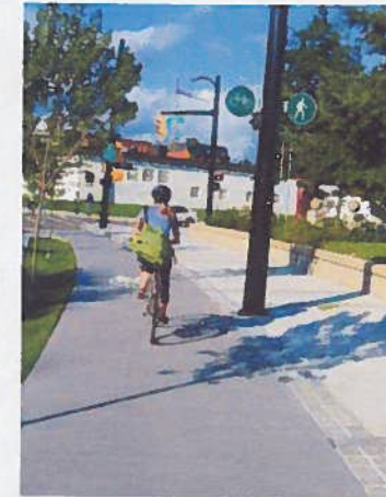
Another off road option which may be perceived as a being safer by less experienced riders is the shared use path with separate bike and pedestrian zones, differentiated by surface design, color, and/or pavement markings.
