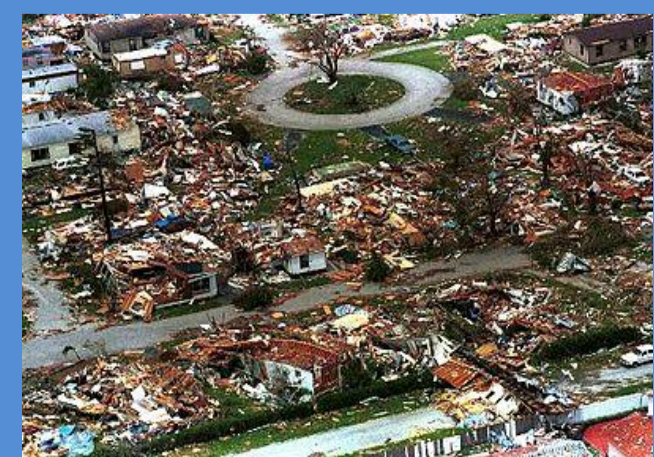
Damage in South Dade County, FL. Courtesy Ray Fairall.
