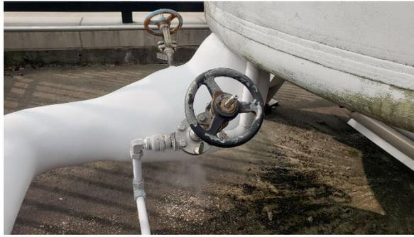
5. Open the small valve one turn on the fill line to begin flow of LN2 in the fill line. It may take a few minutes for the LN2 to start flowing from the end of the line.
