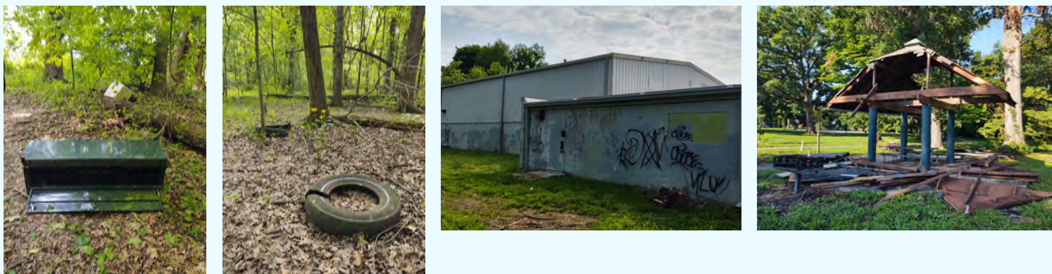
Poor conditions, including trash, graffiti, and deteriorating structures, in Sylvania and Riverside Gardens Parks, 2022. Source: Tony Arnold.
