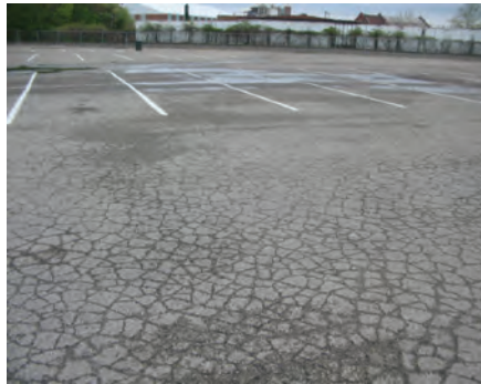
Photos showing the run-off near Old Eastern Parkway and the damaged surface of Parking Lot #1.
