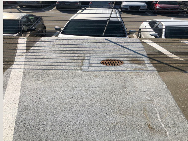
TRAFFIC COATING AND INSTALLATION OF NEW DRAINS
