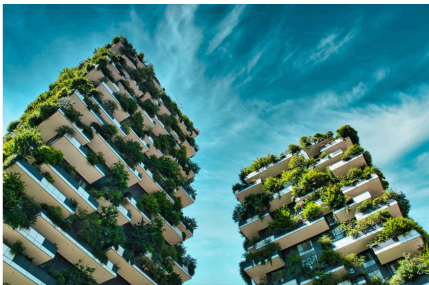
The dual-tower Bosco Verticale in Milan houses more plants and trees than human residents. (Credit: Balazs Sebok/Alamy)
