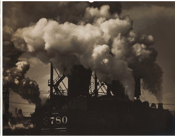
Figure 8 Steel and Smoke
