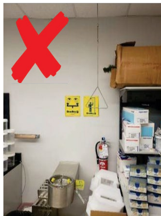
Blocked safety shower obstructed by items
