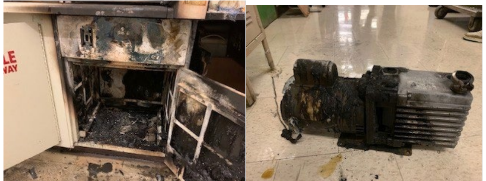
Cabinet damaged by explosion caused by ignition of concentrated ethyl ether vapor from improperly vented vacuum pump exhaust. Ignition source likely electrical switch on motor or fan.
