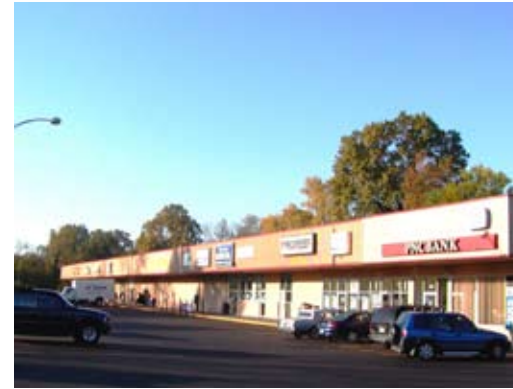
French Plaza, off of Amy Avenue, is representative of existing uses in a “Commerical District”
