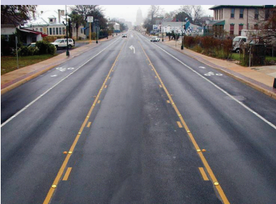
Figure 5-2: Typical 4-lane roadway reconfigured with a “road diet”.
