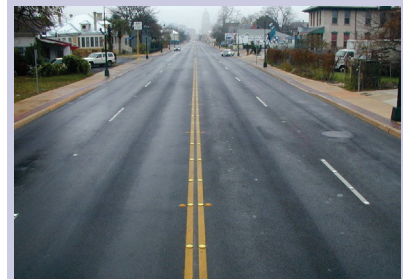
Figure 5-1: Typical 4-lane roadway.
