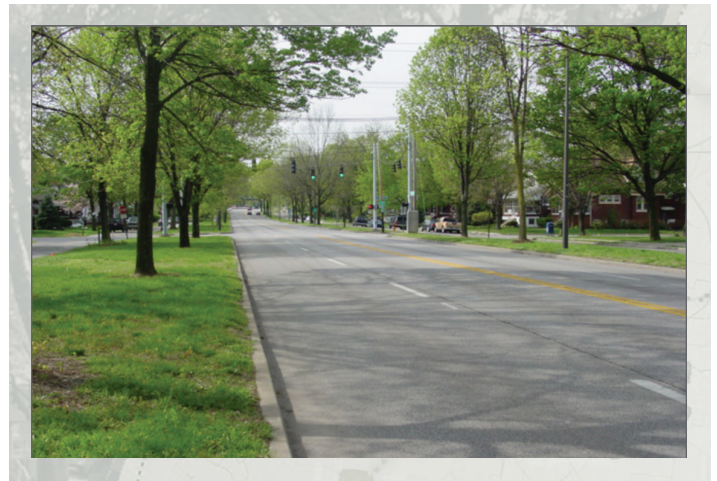
Figure 4-35: Southern Parkway between Wayside Park and Florence Avenue.
