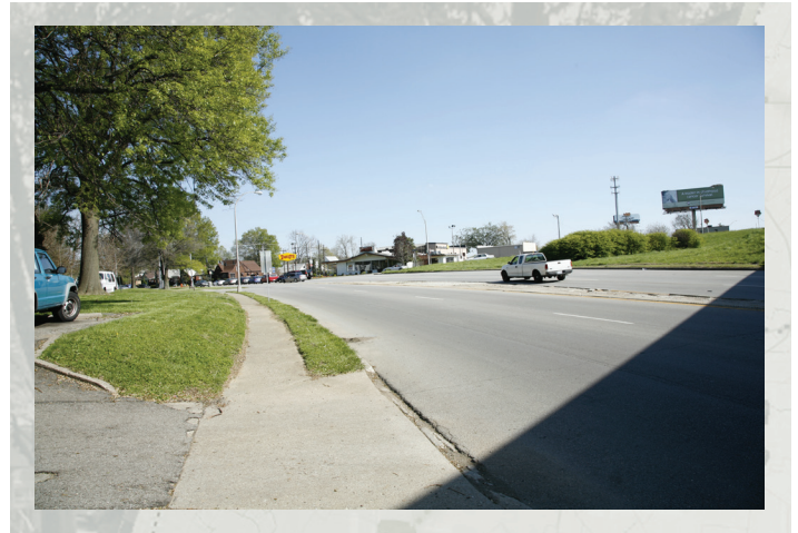
Figure 4-84: Eastern Parkway at Crittenden Drive.
