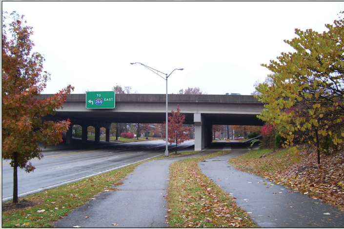
Figure 4-37: Intersection of Interstate 264 and Southern Parkway.
