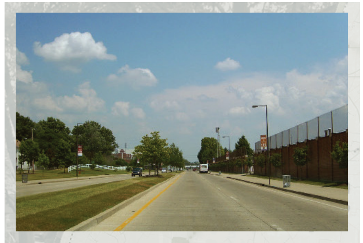
Figure 4-80: Central Avenue at Churchill Downs.
