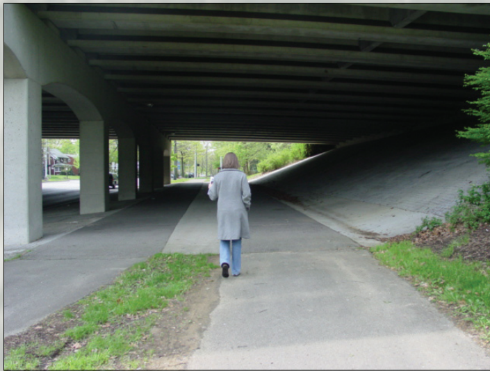
Figure 4-38: Path under Interstate 264 along Southern Parkway.
