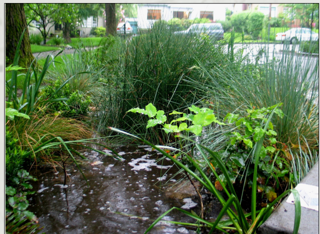
Retaining stormwater runoff
