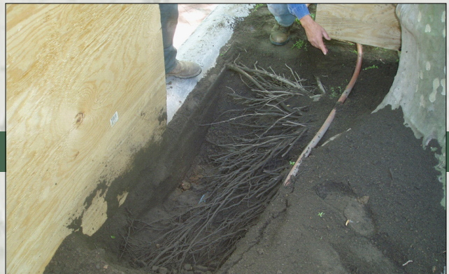
Air spading safely removes soil from tree roots
