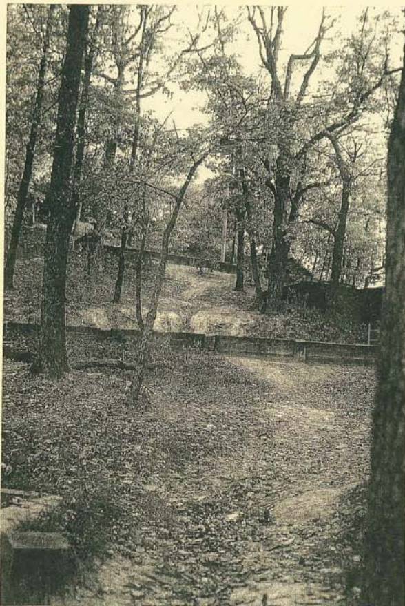
Erosion at steps to the Northern Overlook. (PDR Engineers, 1992)
