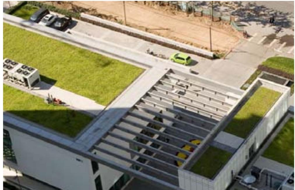
Example of green roof technology applied to an industrial structure.
