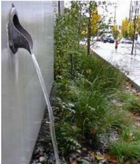
Filtering roof draining before it reaches the municipal storm sewer system improves water quality.
