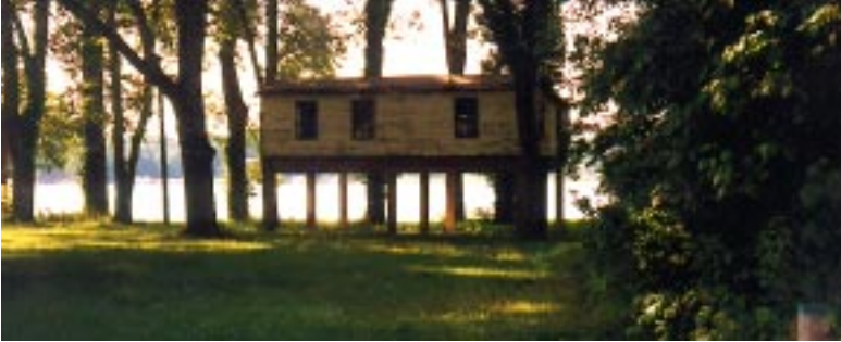
Cottage in the 100-year floodplain.
