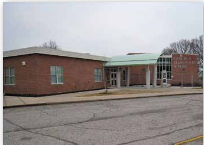
New entryway at Cane Run Elementary School, Louisville, Kentucky
