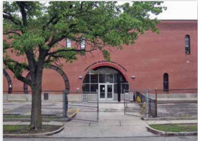
Current entryway to Portland Elementary School, Louisville, Kentucky
