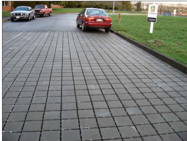
Grid blocks allow water from rain events to soak into the underlying soil. (Photo: U.S. Environmental Protection Agency)
