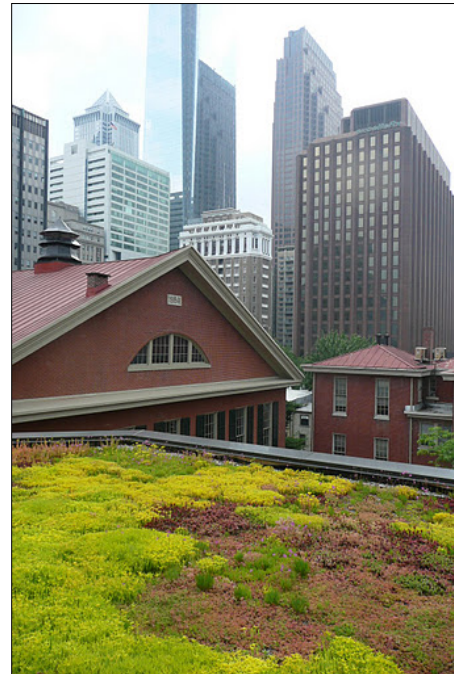
Green roof. (Photo: U.S. Environmental Protection Agency)
