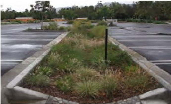
Bio-retention (rain garden) installation. Source: Mid-South Regional Greenprint Vision Plan, 2013
