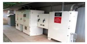
**Figure 9. String inverter** Source: NREL PIX 07985
