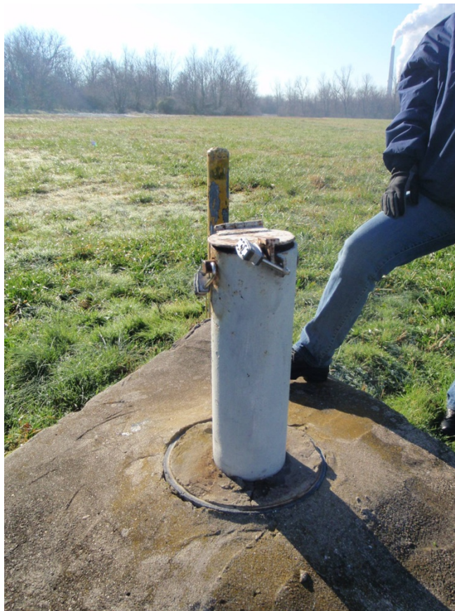
Ground water monitoring well near the cap along Ohio River. The well is securely locked.
