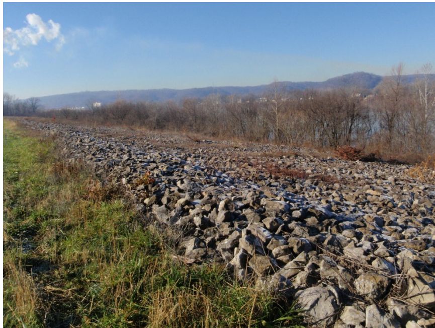
Rip rap between the cap and the Ohio River.
