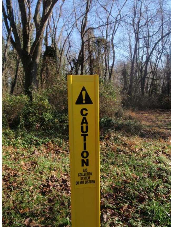
Signs clearly marking the gas extraction system.
