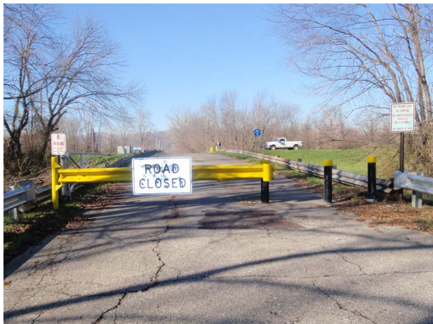
Entrance from Lee's Lane. Gate is locked and maintained by MSD.
