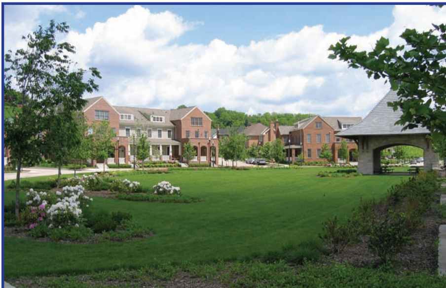
Summerset at Frick Park in Pittsburgh, Pennsylvania, built on a former brownfield.
