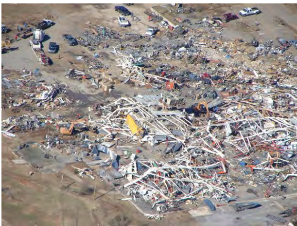
Businesses across Arkansas were damaged or destroyed by the 2008 tornadoes. This boat building business in the city of Clinton, in north central Arkansas, was particularly hard-hit. Credit: Vaughan Wingfield, UALR Institute for Economic Advancement.
