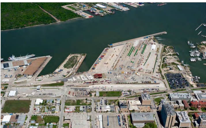
The Port of Galveston’s east end revitalization project will provide additional cargo storage and better intermodal connections to the surrounding region. Credit: H-GAC.
