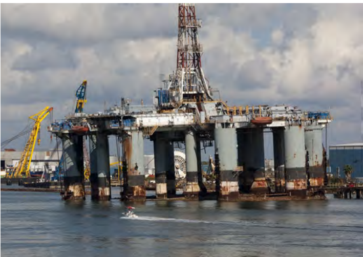
This oil platform was damaged beyond repair when Ike passed through the Gulf of Mexico. Credit: Flickr user Dean Terry.
