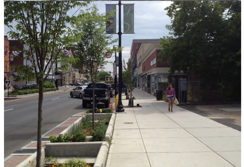
North Street before (top) and after (bottom) rain garden retrofits.
