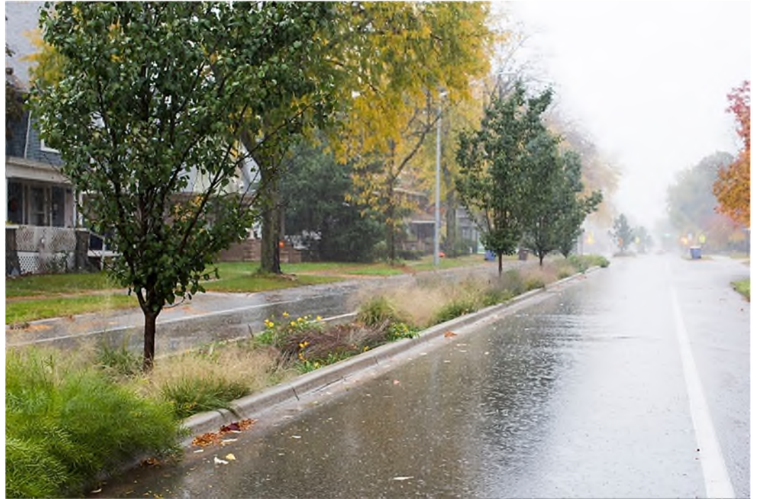
One of seven bioretention islands on Plainfield Avenue. Photo credit: David Kidd, Governing Magazine.
