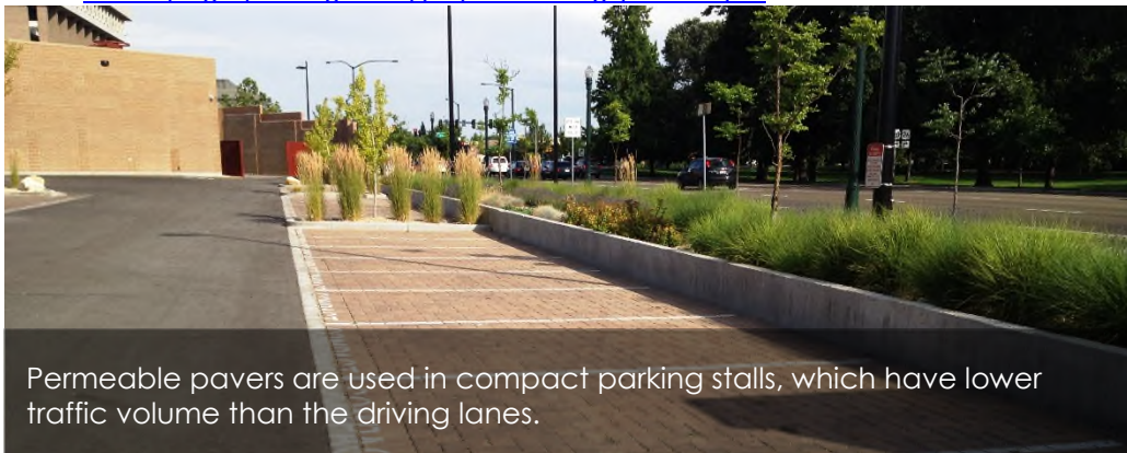
A bioretention area treats runoff from the parking surface and is planted with low-maintenance vegetation.
