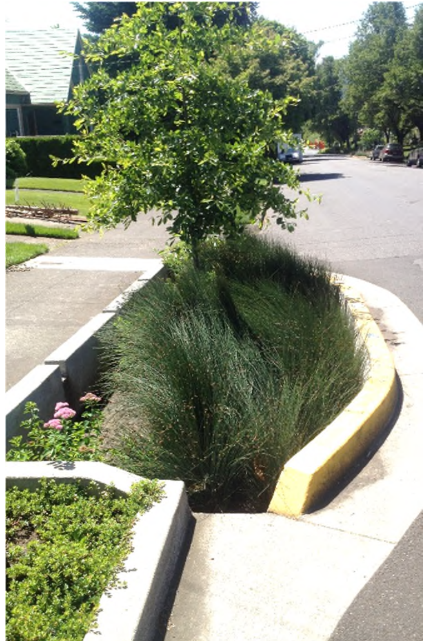
This bioretention bump-out captures runoff and slows traffic on a road frequented by cyclists and pedestrians.
