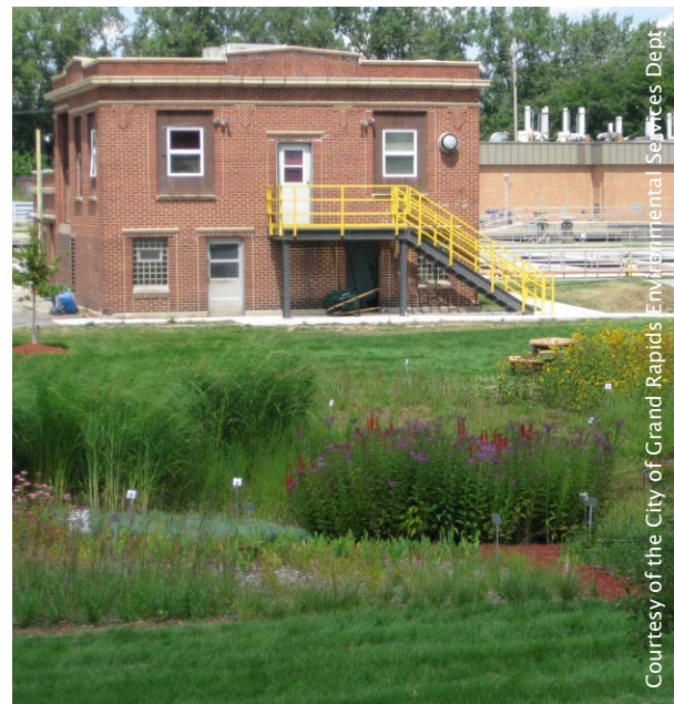
Exhibit 22. River of Dreams rain garden, Grand Rapids, Michigan. The city of Grand Rapids’ Environmental Services Department installed a rain garden on an old tank site that is able to divert 1.5 million gallons of untreated stormwater from the Grand River annually.
