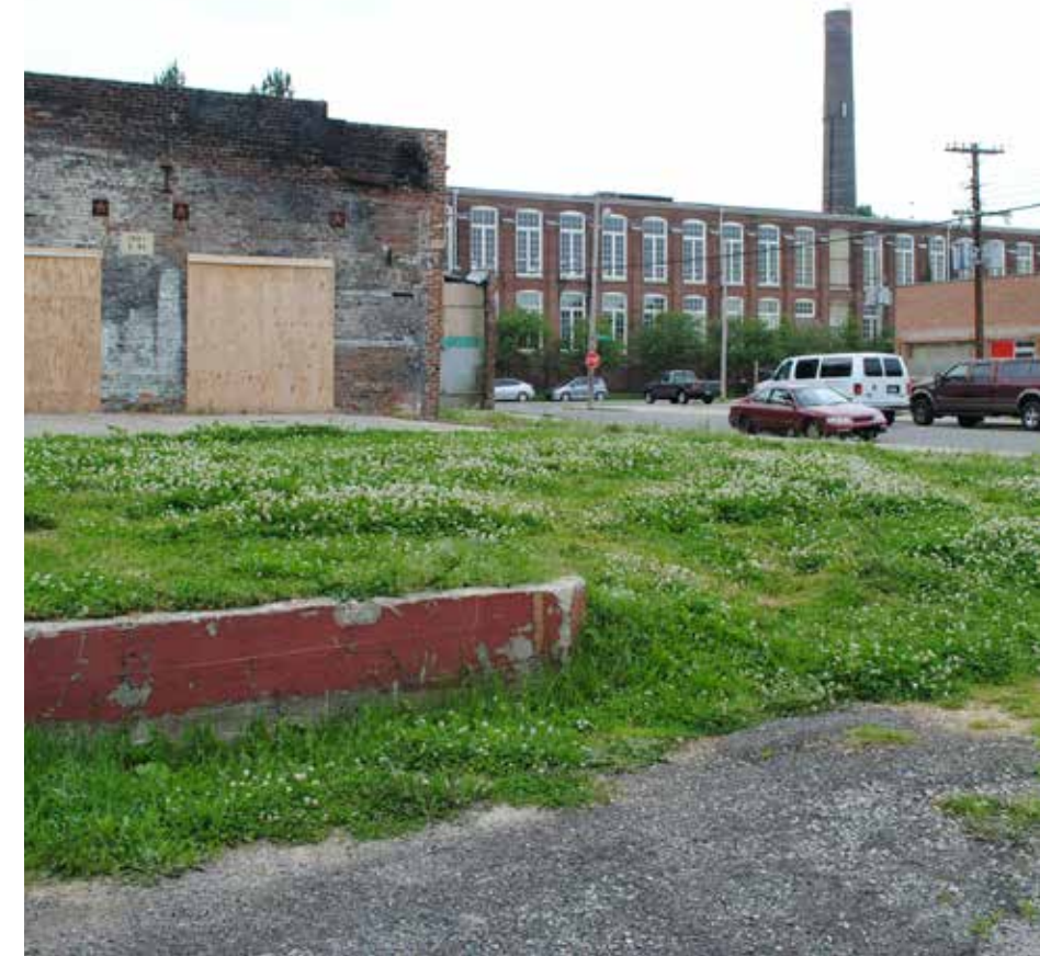
SITE D: WASTE TRANSFER STATION
