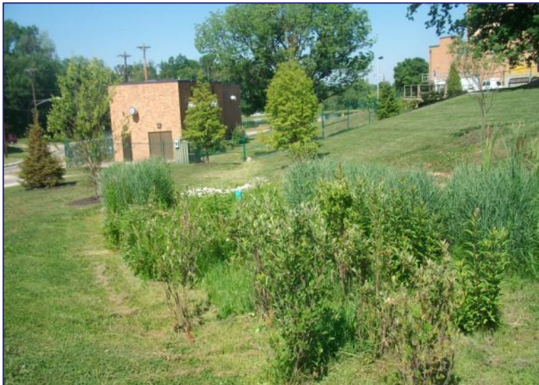
Memorial Parkway Biofiltration Swales – Ft. Thomas
