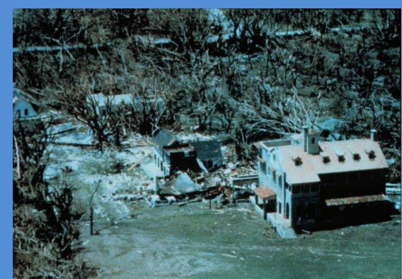
Deering Estate in FL. Water marks from storm surge. Courtesy NOAA.
