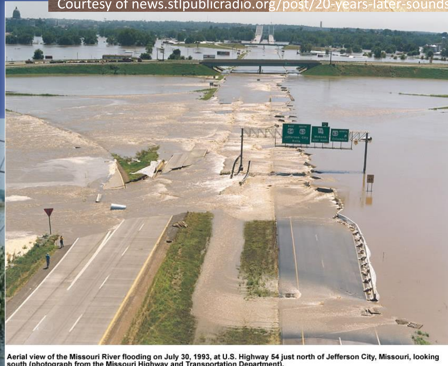
Aerial view of the Missouri River flooding on July 30, 1993, at U.S. Highway 54 just north of Jefferson City, Missouri, looking south (photograph from the Missouri Highway and Transportation Department).
