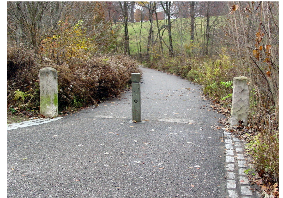
Metro Parks Standard Bollards - Steel and Limestone
