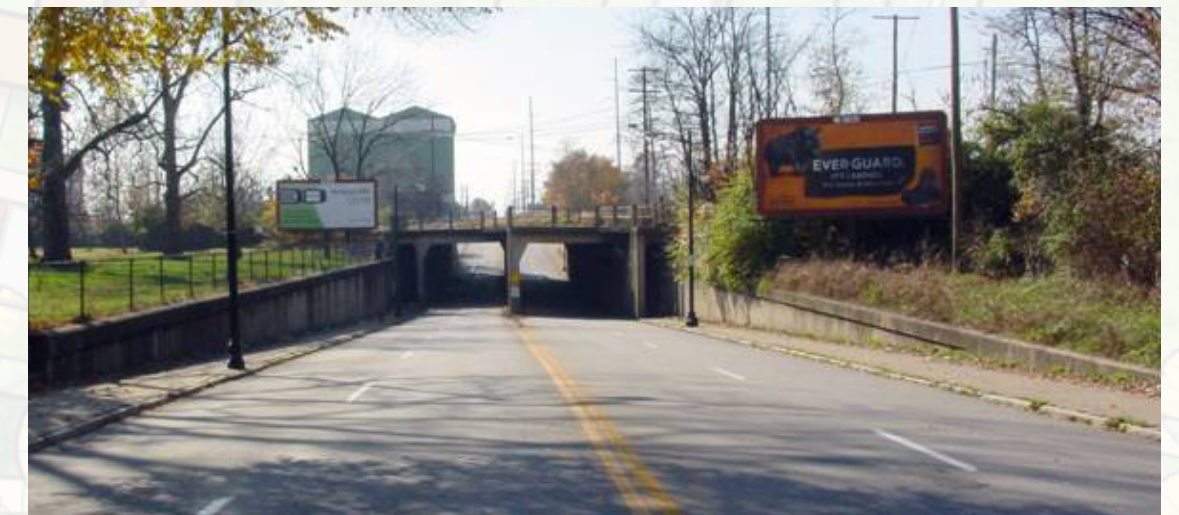
Cleanup adjacent right-of-way; add tree plantings, remove bilboards and establish new street tree plantings.
