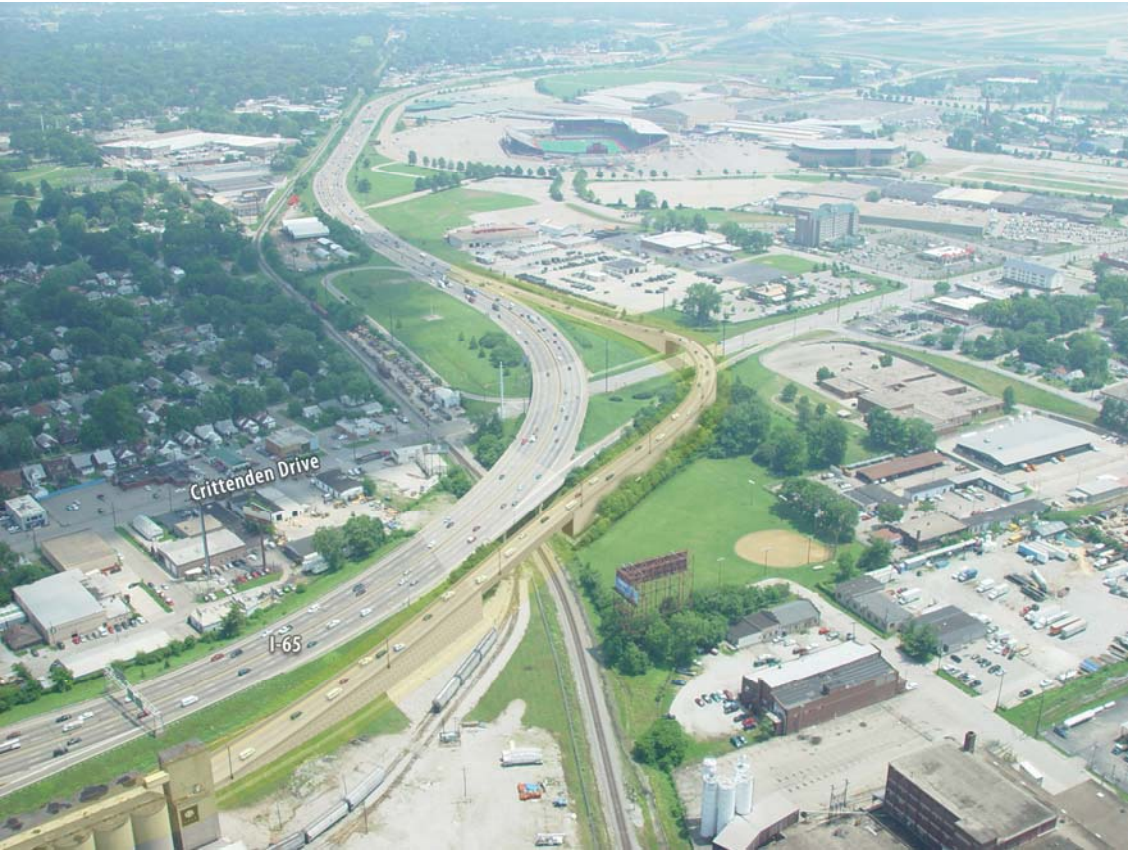
FIGURE ES7A – SIMULATION SHOWING POSSIBLE NEW RAMP FROM EASTERN PARKWAY TO SOUTHBOUND I-65
