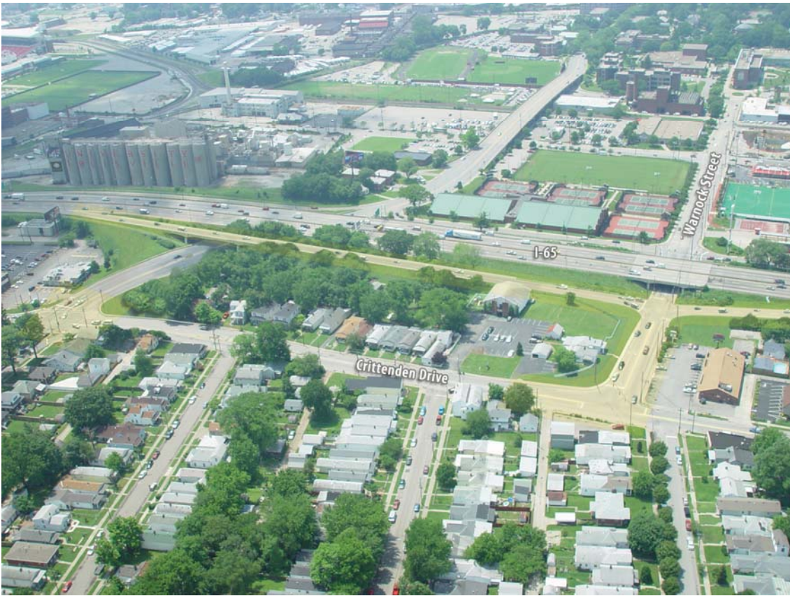
FIGURE ES9A – SIMULATION SHOWING POSSIBLE NEW EXIT RAMP FROM NORTHBOUND I-65 TO WARNOCK STREET
