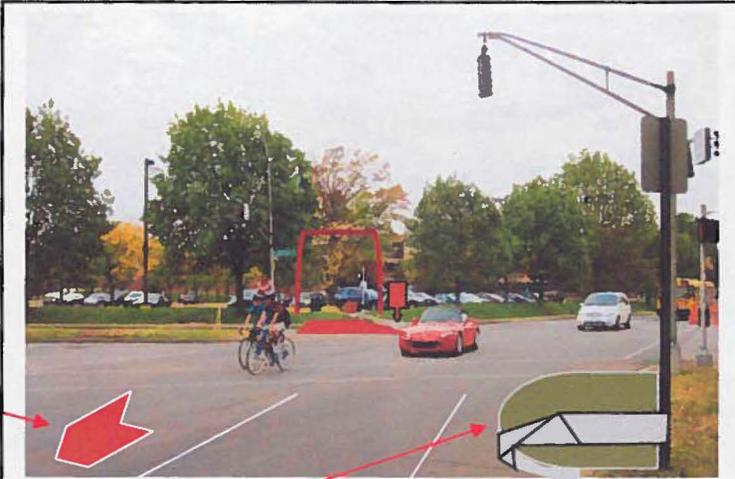
Installing curb bumps into parking lanes reduces crossing distances (and times) for pedestrians; increases safety.
