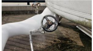
5. Open the small valve one turn on the fill line to begin flow of LN2 in the fill line. It may take a few minutes for the LN2 to start flowing from the end of the line.
