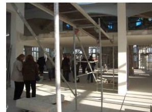
Mosque under construction
