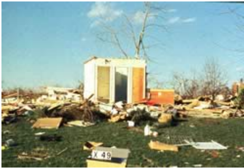
Safe Room remains standing after a tornado destroys the house it was in. The residents were spared from any injuries. Photo from Texas Tech University
