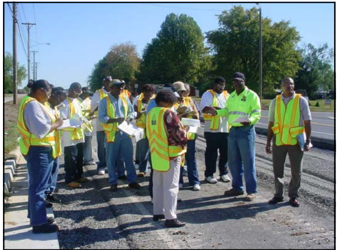
Workforce Development participants visit highway construction site
