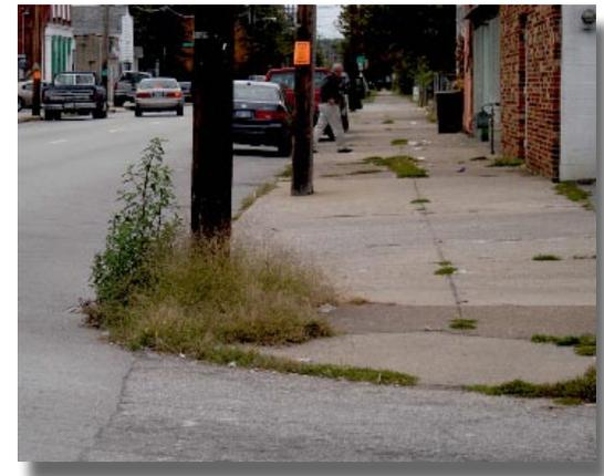
*Most streets in Portland need improved maintenance, pavement and curb replacement or repair, and retrofitting with handicap curb cuts at intersections in order to provide a positive pedestrian experience throughout the neighborhood.*
