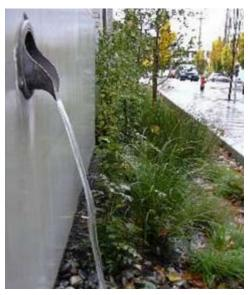
Filtering roof draining before it reaches the municipal storm sewer sytem improves water quality.
