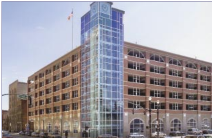
First and Main Garage
