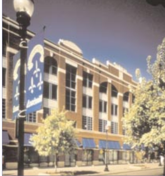
Fifth Street Garage
