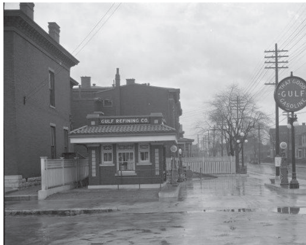
BRECKINRIDGE AVENUE, SMOKETOWN
