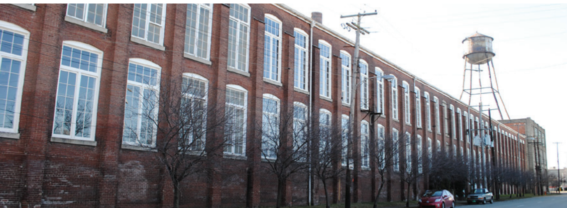
HOPE WORSTED MILLS ORIGINAL STRUCTURE
