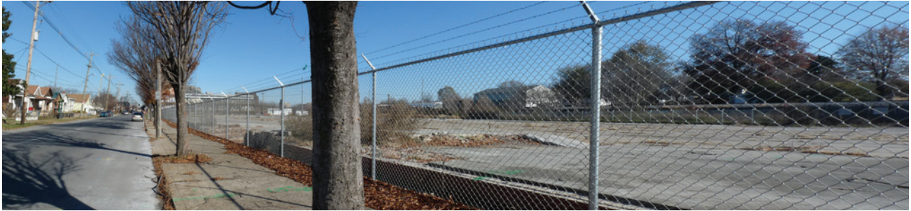
EXISTING CONDITIONS OF THE MSD BASIN
