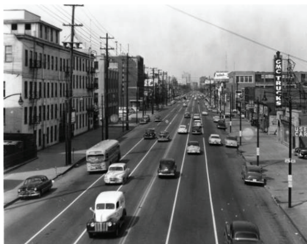
BROADWAY LOOKING WEST FROM THE SHORT LINE VIADUCT
