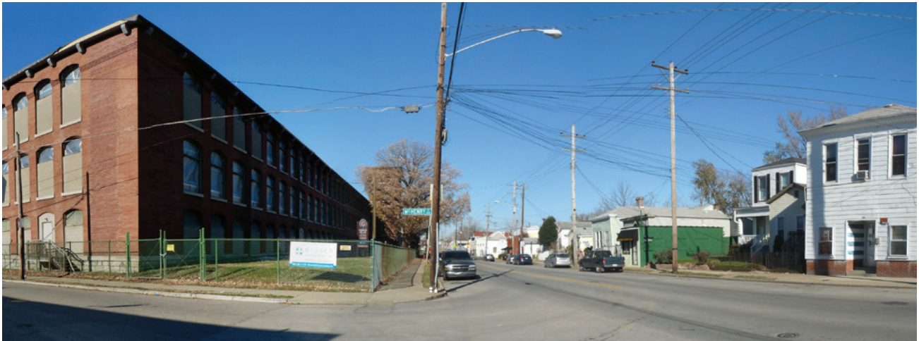
EXISTING CONDITIONS OF GOSS AVENUE
