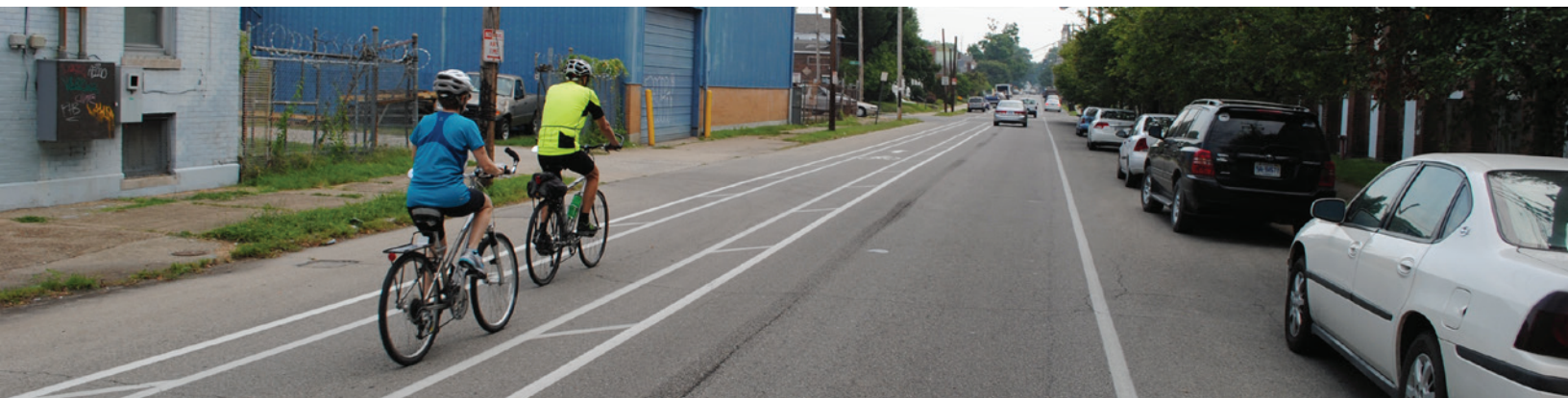
EXISTING BIKE LANE ON KENTUCKY STREET
