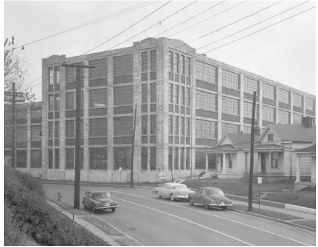
EXISTING BRADFORD MILLS
