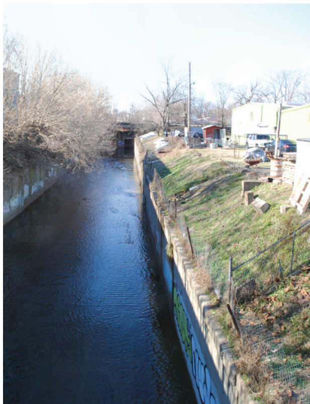
CURRENT CONDITION OF BEARGRASS CREEK
